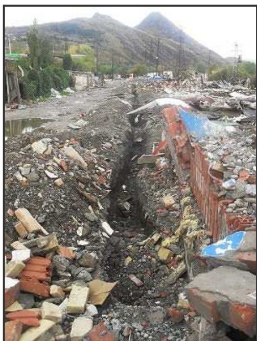
Trench dug by children to extract electrical cable from toxic ground in Cesmin Lug camps
